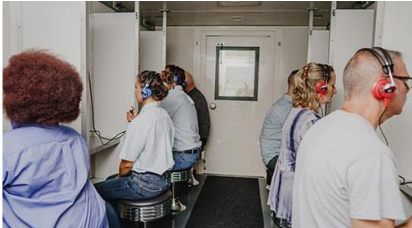
Fixed installation of sound booths
